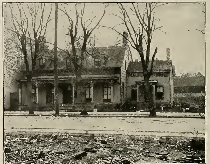
The Michael Prior House, Bergen Avenue near Duncan Avenue
